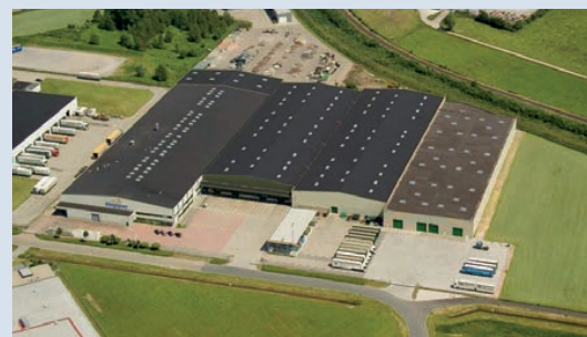
Kingspan Insulation Winterswijk, Niederlande
