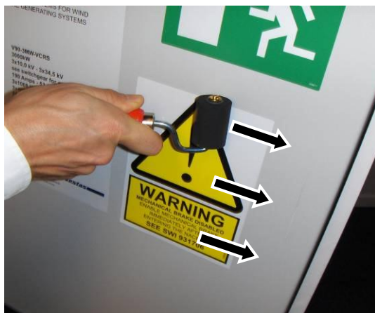
Figure 12-7: Rolling towards right-hand side
