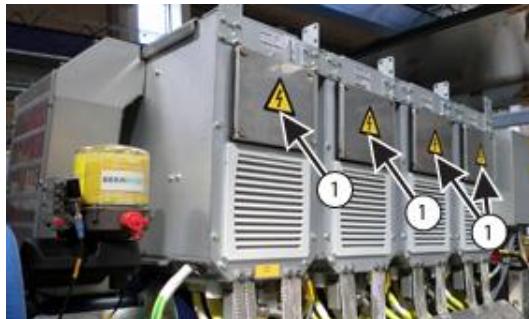
Figure 16-14: GIM units facing the nacelle control units
