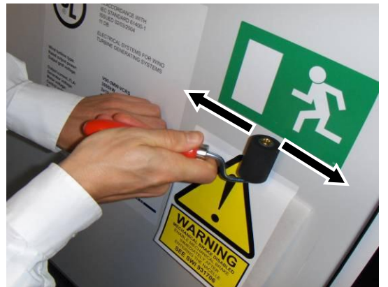
Figure 12-4: Using a roller to make the sign stick
